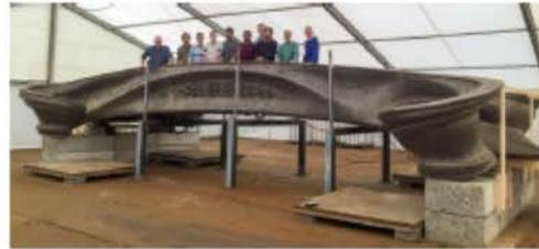
AM metal bridge, printed by mx3d ([www.mx3d.com](http://www.mx3d.com)) Picture courtesy of M2i ([www.m2i.nl](http://www.m2i.nl))
